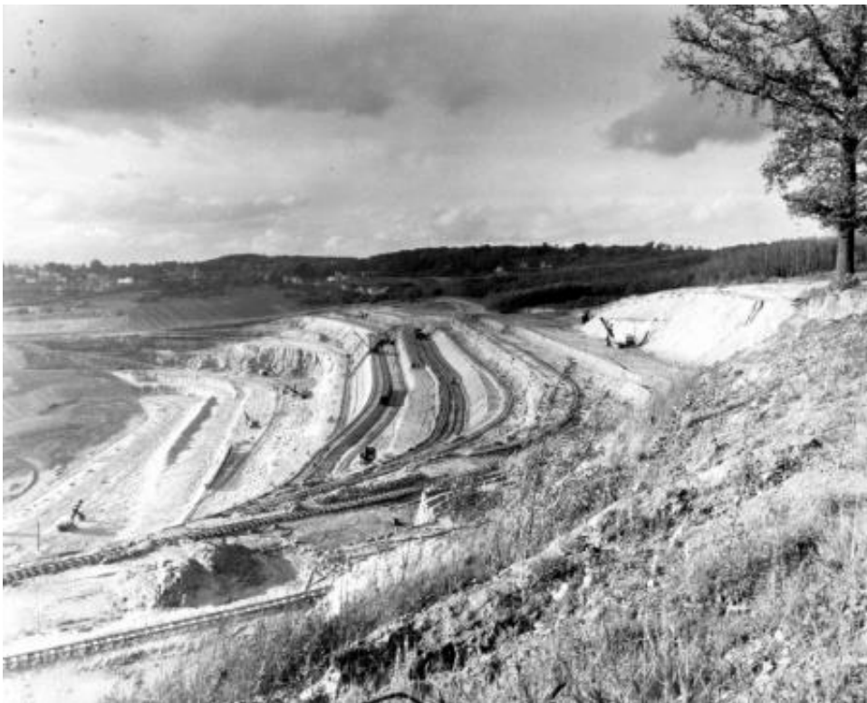
The Lambert quarry in the 1950s. Mechanisation accelerates production. Benches mark the separations between the various geological strata. Narrow-gauge diesel locomotives and wagons run on the tracks laid on each bench, under each cutting face. Musée du Plâtre collection.
